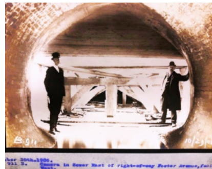
1906: Foster Avenue Sewer Under Brighton Tracks
