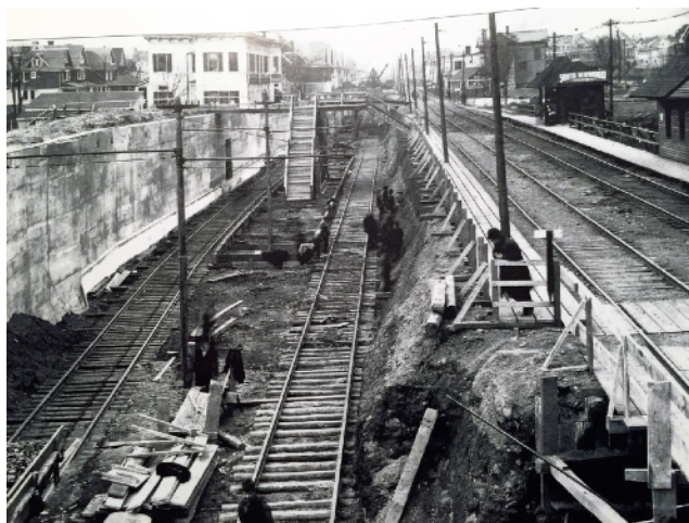
Retaining Wall Construction at Newkirk Avenue in 1906
